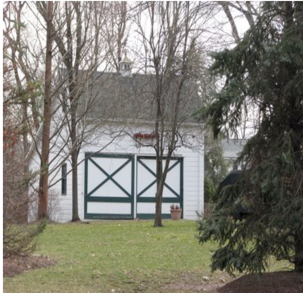
Barn located at 289 West Street
