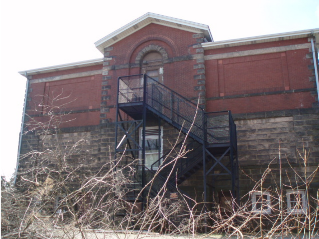
View of the rear (west) façade
