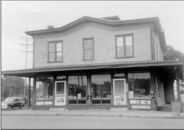
The John Henry Stevens Store, as it appeared before it was demolished in 1957, displayed two typical turn-of-the-century storefronts with large amounts of glass.
