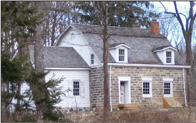
The main section of the Walter Parsells House has the sturdy sandstone first-story walls characteristic of the early stone houses.
