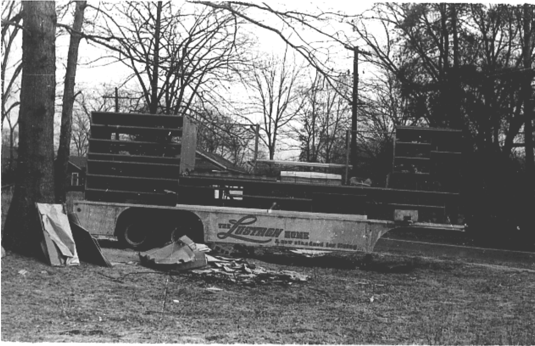
The Lustron Truck at the Harold Hess property 1950 – this truck could carry all of the components for building the house
